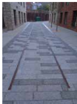
The surviving tramlines in the new footpath in Magdalen Street
