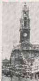
COLCHESTER TOWN HALL AND VICTORIA TOWER
