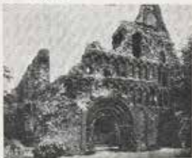
ST. BOTOLPH'S PRIORY CHURCH
