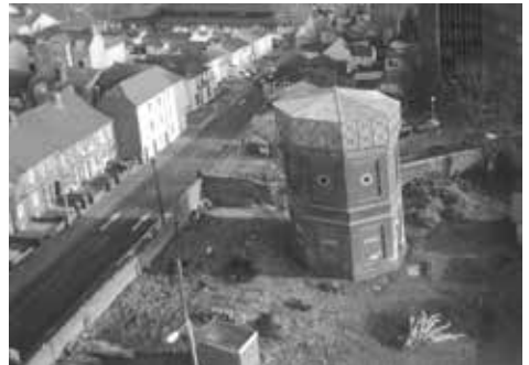
The original Bath House before the building work
