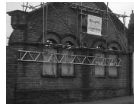
Surviving frontage, Military Road
