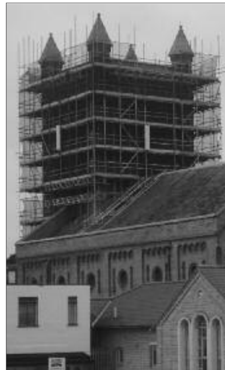
St Botolph's Church with scaffolding
