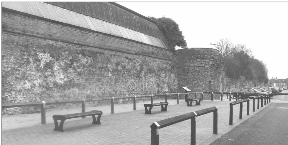
The newly landscaped Roman Wall in Priors Street
