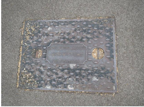
Appleton Moss builders Colchester
