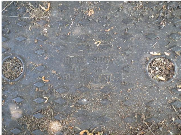
Nock Bros builders Colchester
